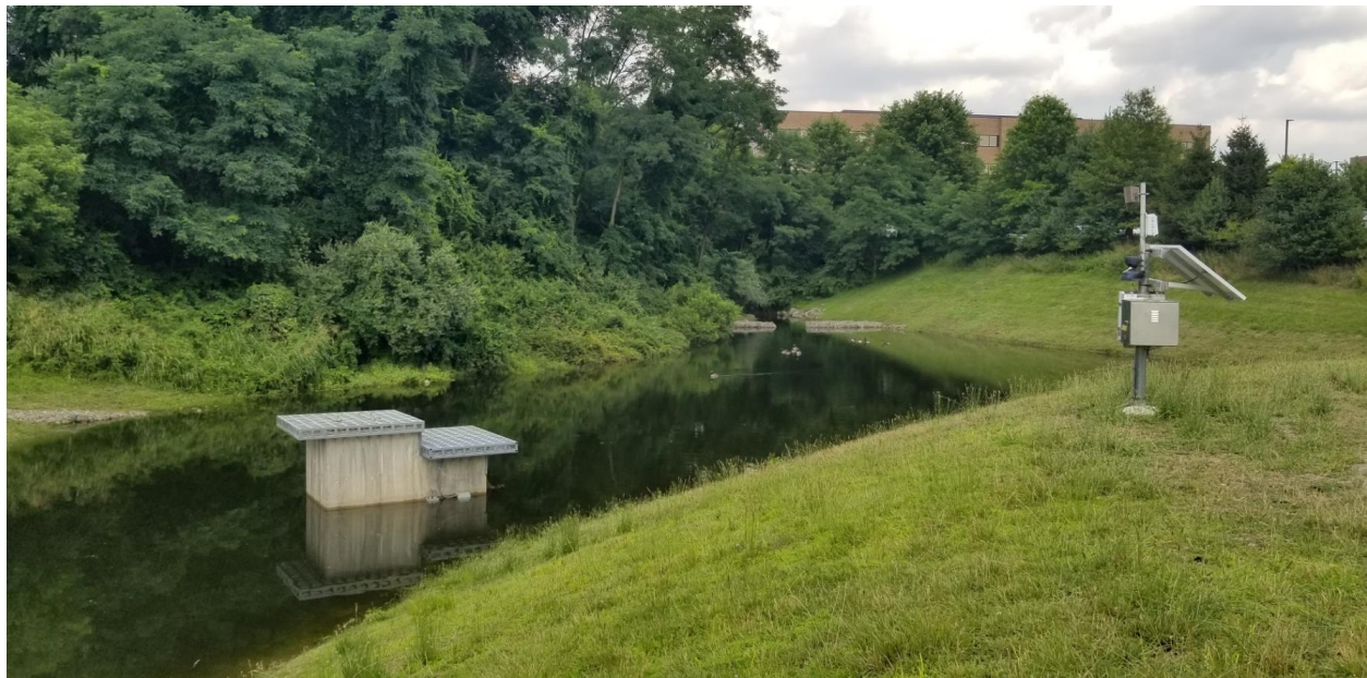
Image: WalMart pond after 2018 retrofit
