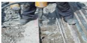
Pavement Removal
